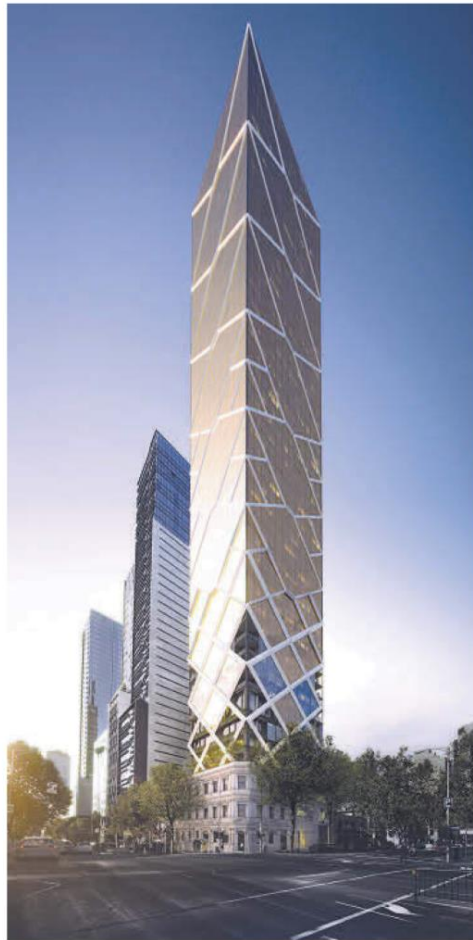
Paragon comprises 227 luxury apartments in Melbourne's CBD
